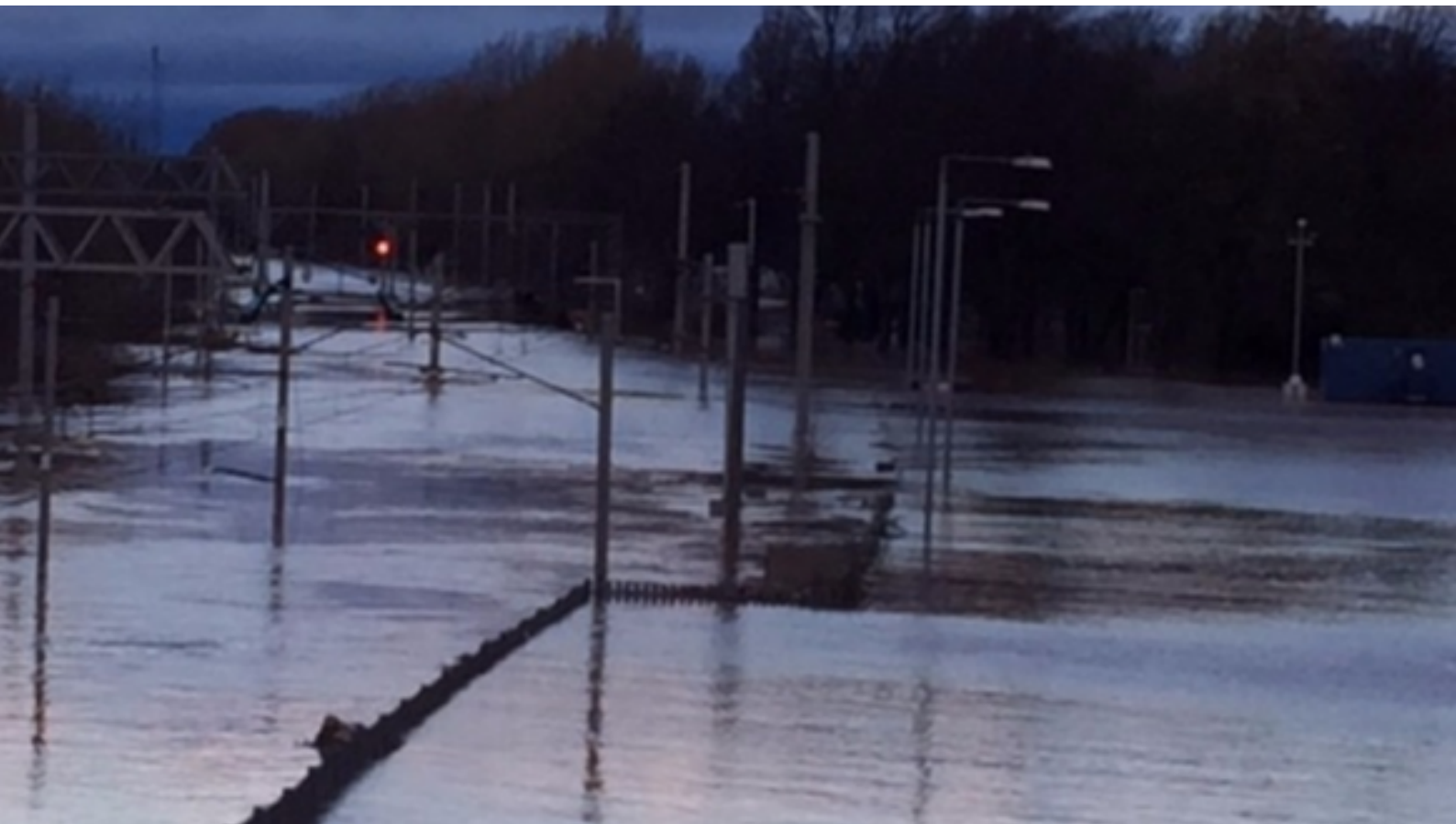
The West Coast Main Line 'under 8ft of water' at Carlisle, January 2016 (Source: ITV)
