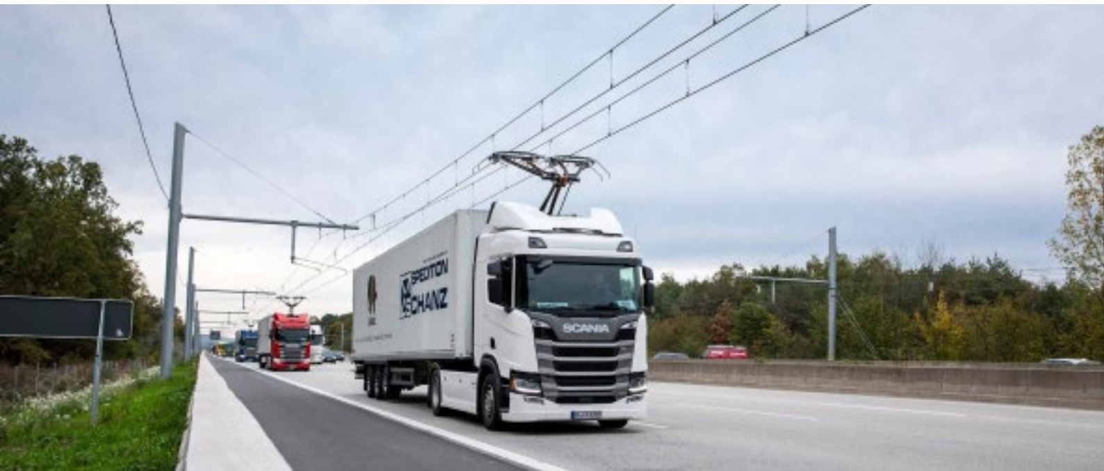
Swedish example of electrified HGV system
