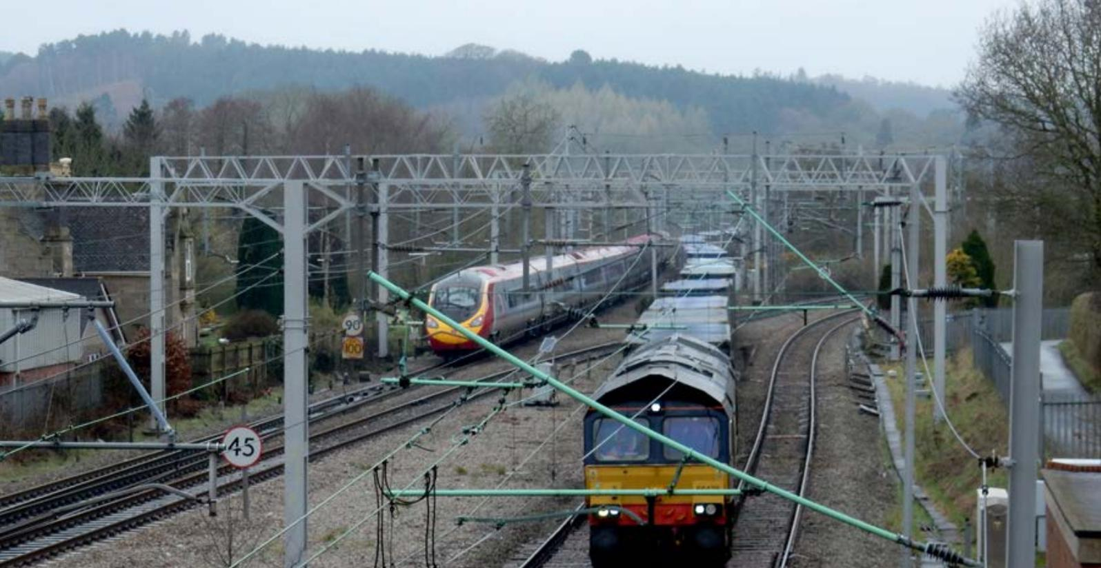
Colwich Junction – speed and capacity constraints where four tracks become two.
