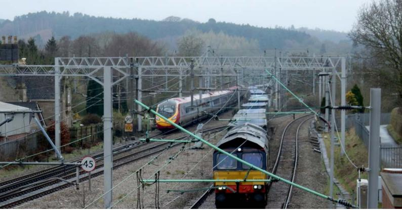
Colwich Junction – speed and capacity constraints where four tracks become two. Photo: Greengauge 21, 2015
