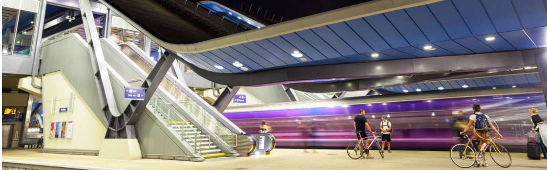
Figure 2.2. Reading's new station. (courtesy of Bechtel / Network Rail)
